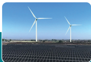
Hybrid Power Plant
