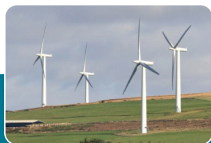
Wind Power Plant
