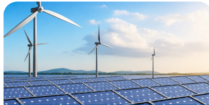
400+ MW Hybrid Power Plant
