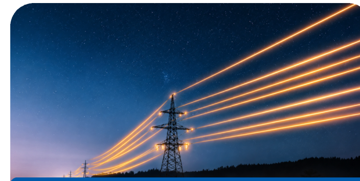
Upto 400KV / 400+ km Transmission Line
