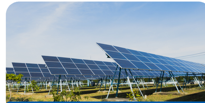
450+ MW Solar ground Mount
